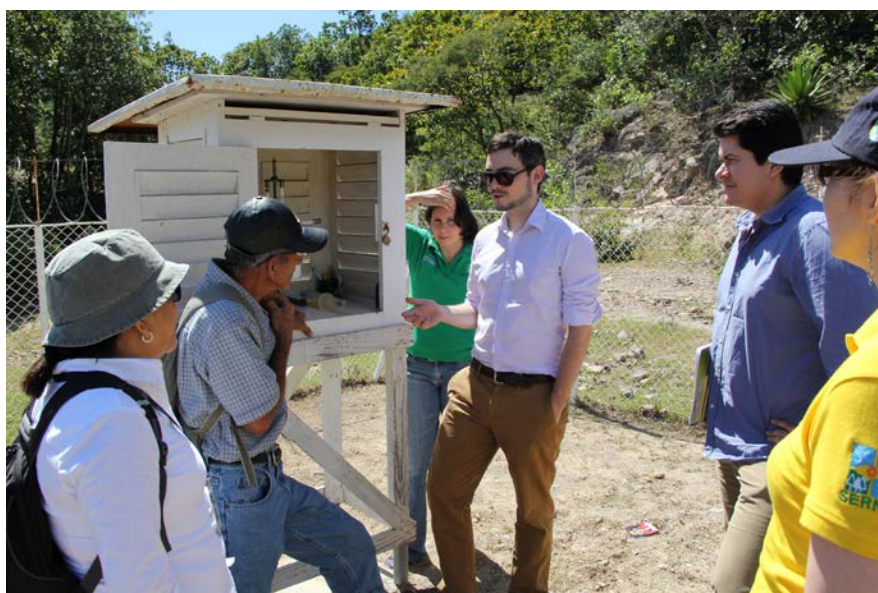
Image 3 – Staff from the mission team discuss the installation of automated weather stations for generation of climate information with system operators
